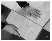
**Cut Palisade tiles** by scoring and snapping with a utility knife (image 6, 7). This method may require sanding the snapped edges.
